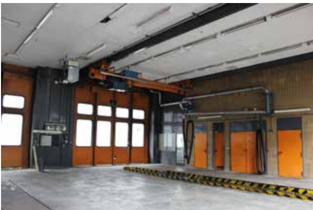
Foto 9: Blick in Werkstatt, Erdgeschoss Annex N2a
