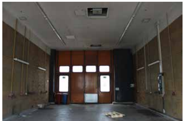
Foto 10: Blick in Werkstatt, Erdgeschoss Annex N2a
