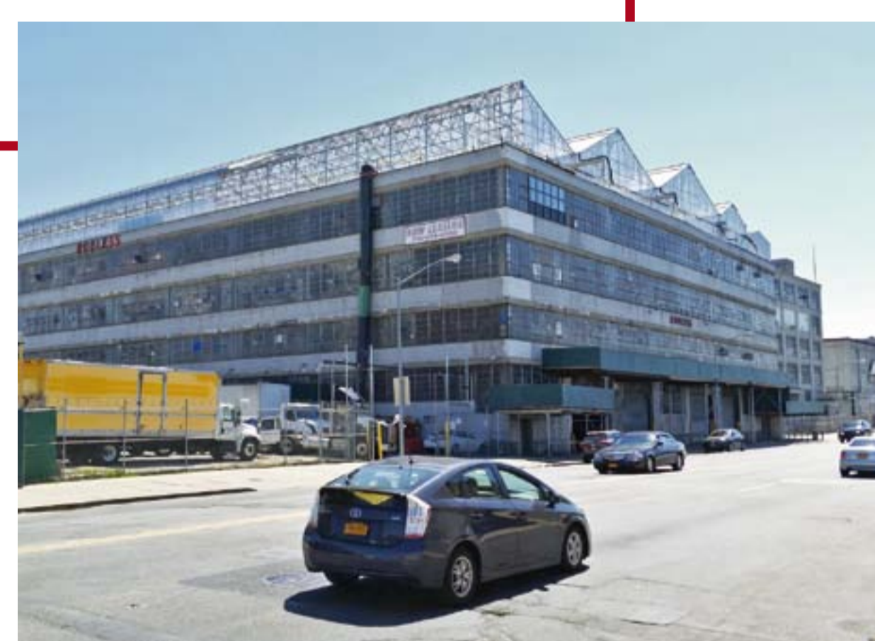
Photo: Matt Green, rooftop greenhouse under construction, flickr.com, CC-BY-SA 2.0
