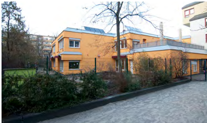
Daycare centre Wolgaster Strasse after renovation
