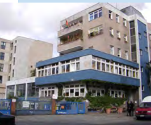
Building before renovation
