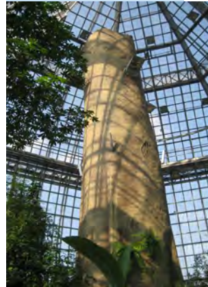
Ventilation towers disguised as tropical trees
