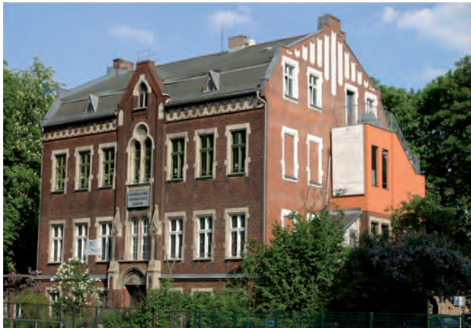
Building before renovation
