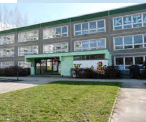
Daycare centre "Akazieninsel" before renovation © Fromm, TraBant GmbH
