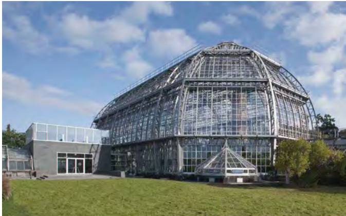
Tropical greenhouse after renovation
