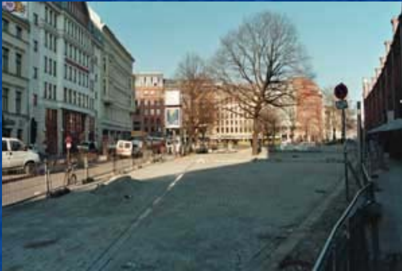
During reconstruction works in 2003
